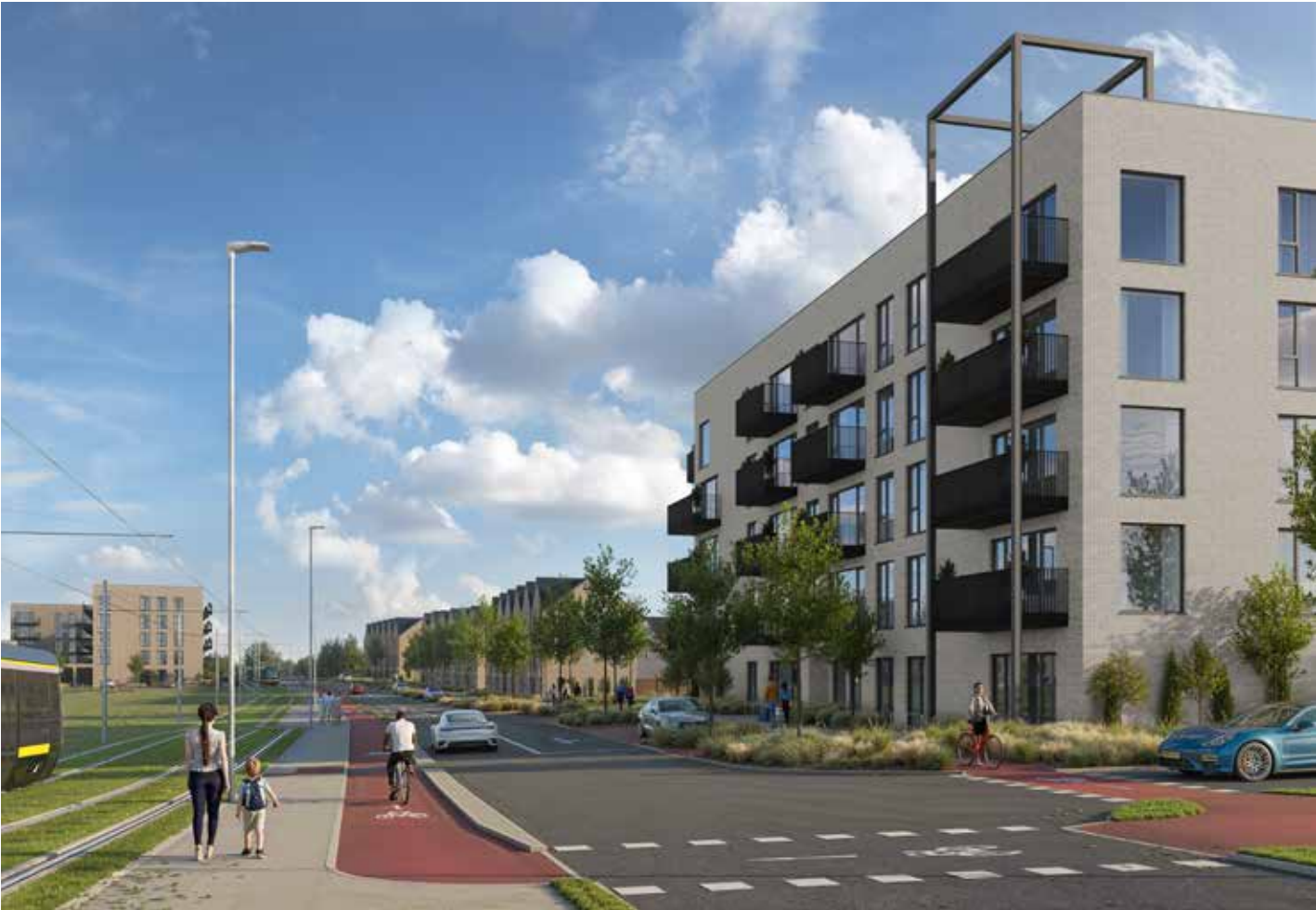
View 6: Block 3 and main N/S road looking south
