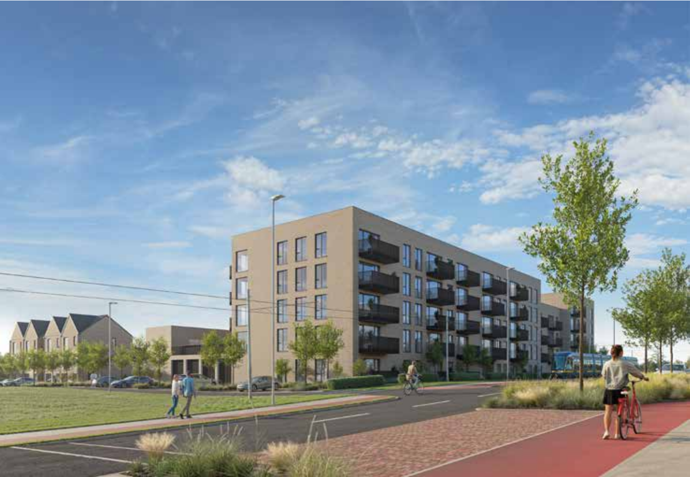
View 4: Primary north-south street, looking south
