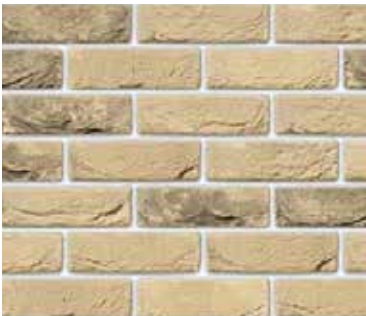
Precedent Image: Buff brick with light grey mortar, from Woodbrook Phase 1
